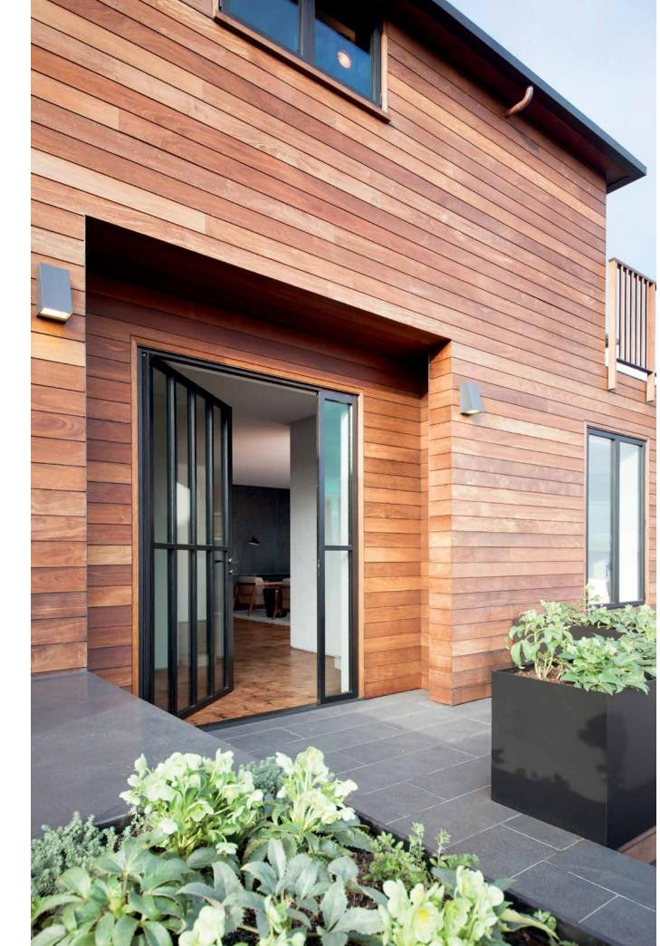
Lundberg clad the residence with horizontal ipe siding that provides texture and an organic feel. The wood frames the entry door, located on the second level, and also acts as a counterpoint to the slate paving and steel planter boxes.
